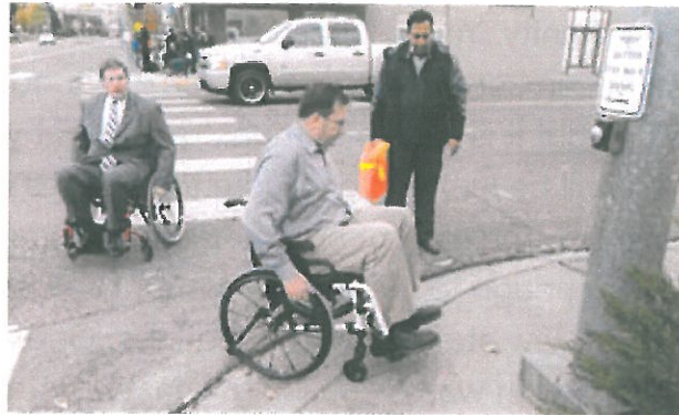
Wheelchair tour with Pasco Mayor and City Engineer getting firsthand experience with substandard ramps.
