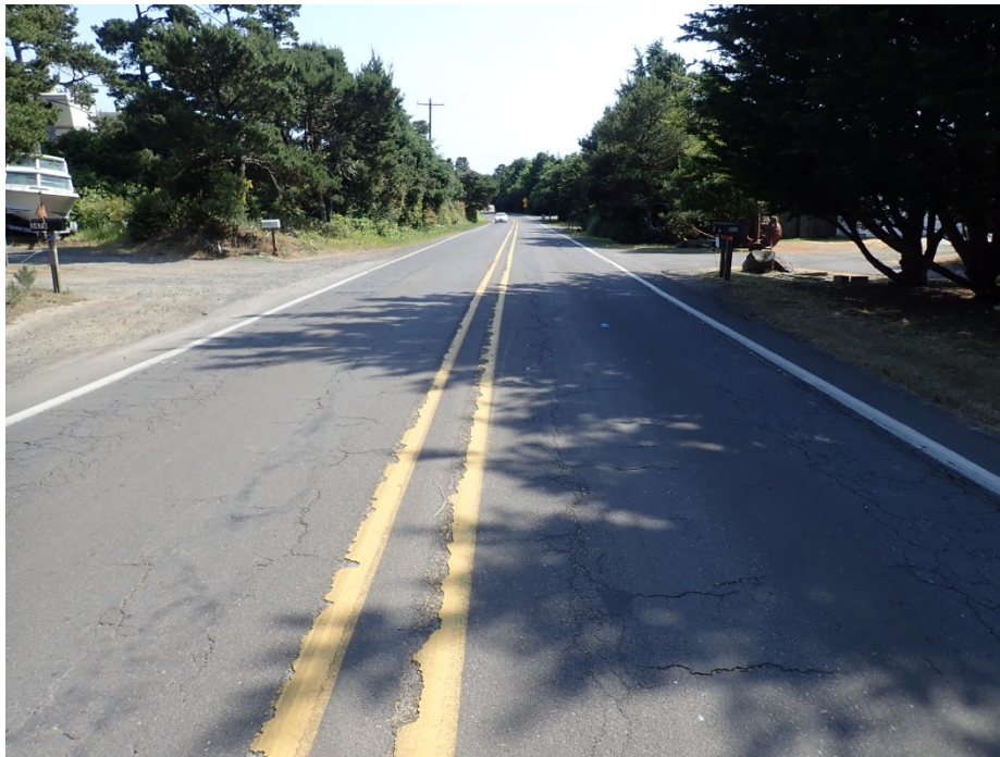
18. Looking south from 350 feet south of 35 th Street.
