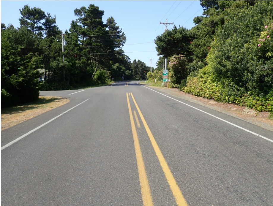
9. Looking north from 100 feet south of Jetty Road.
