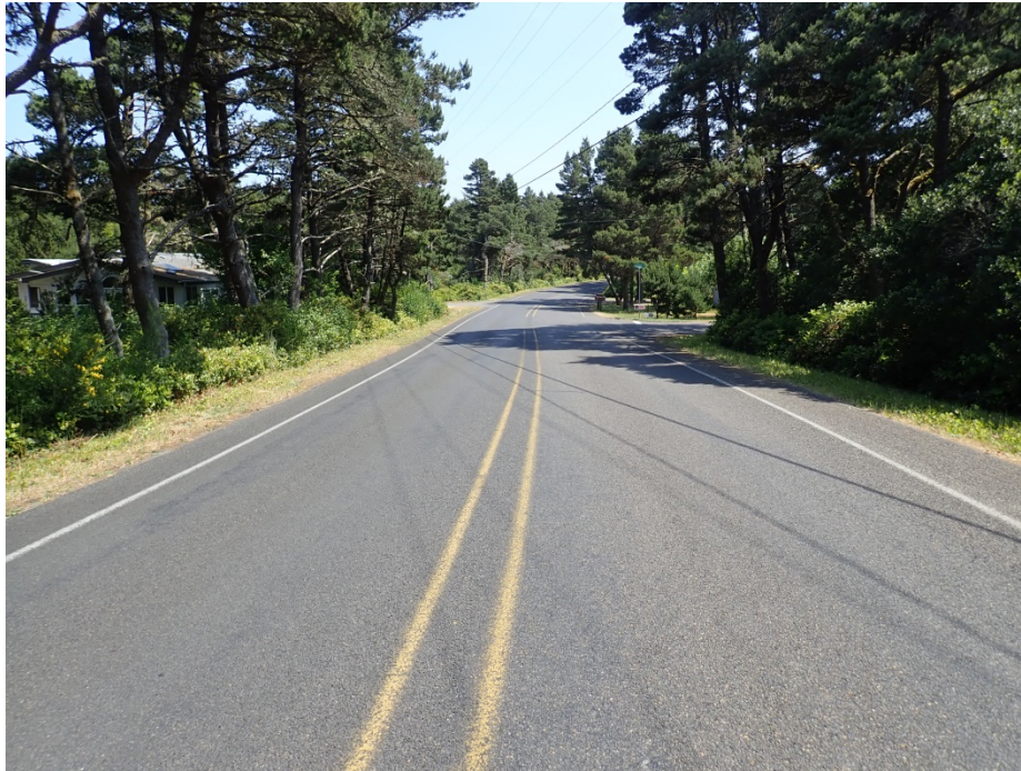
4. Looking south from 125 feet north of Arago Street.
