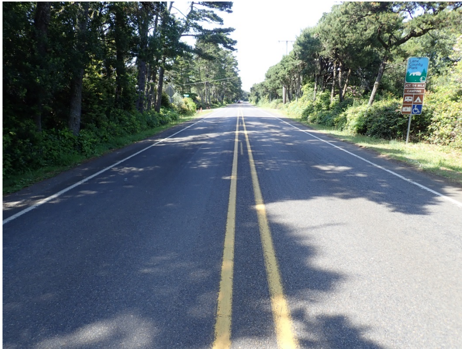
11. Looking north from 100 feet north of Treewood Drive.
