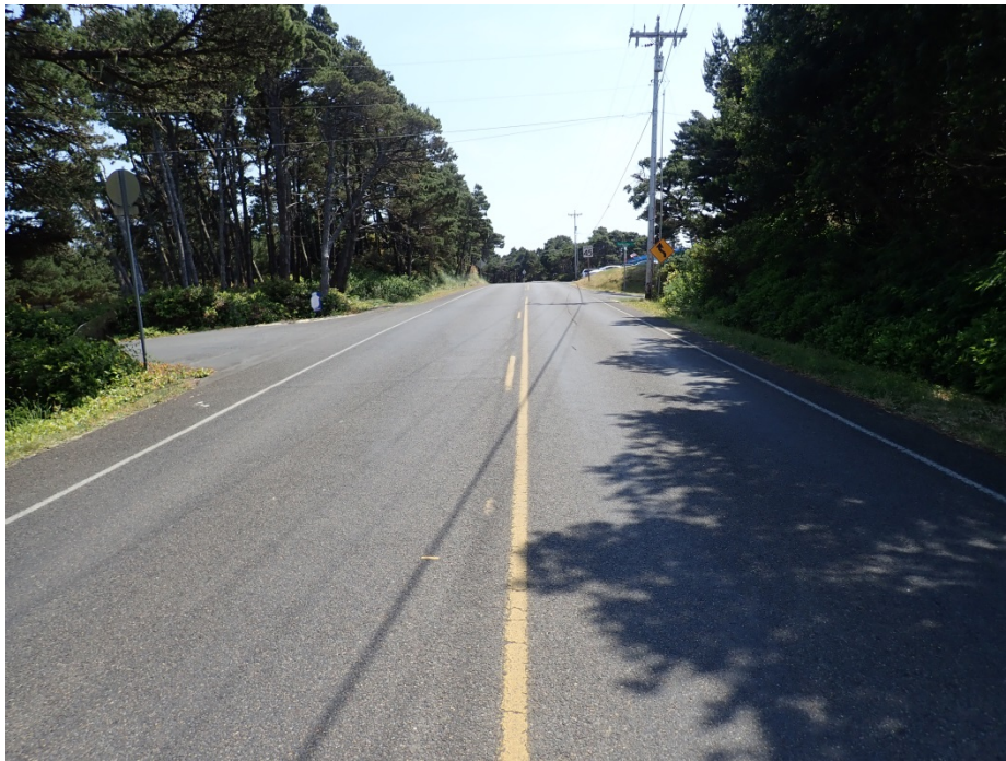
2. Looking south from 150 feet south of Heceta Beach Road.
