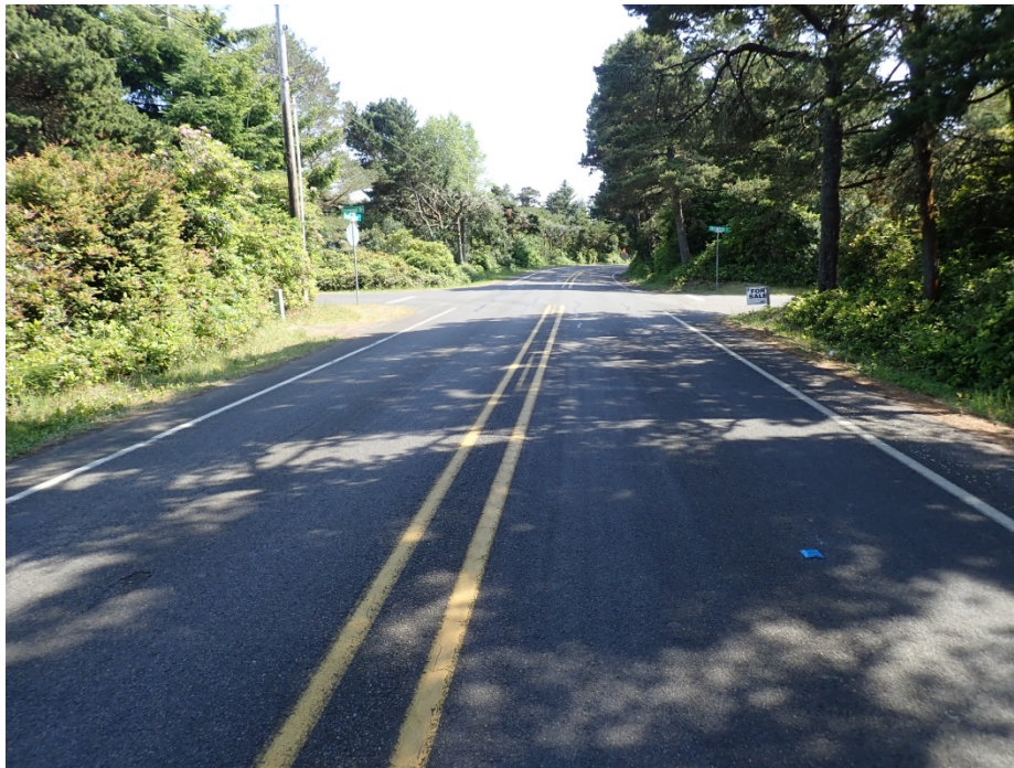
12. Looking south from 100 feet north of Treewood Drive.
