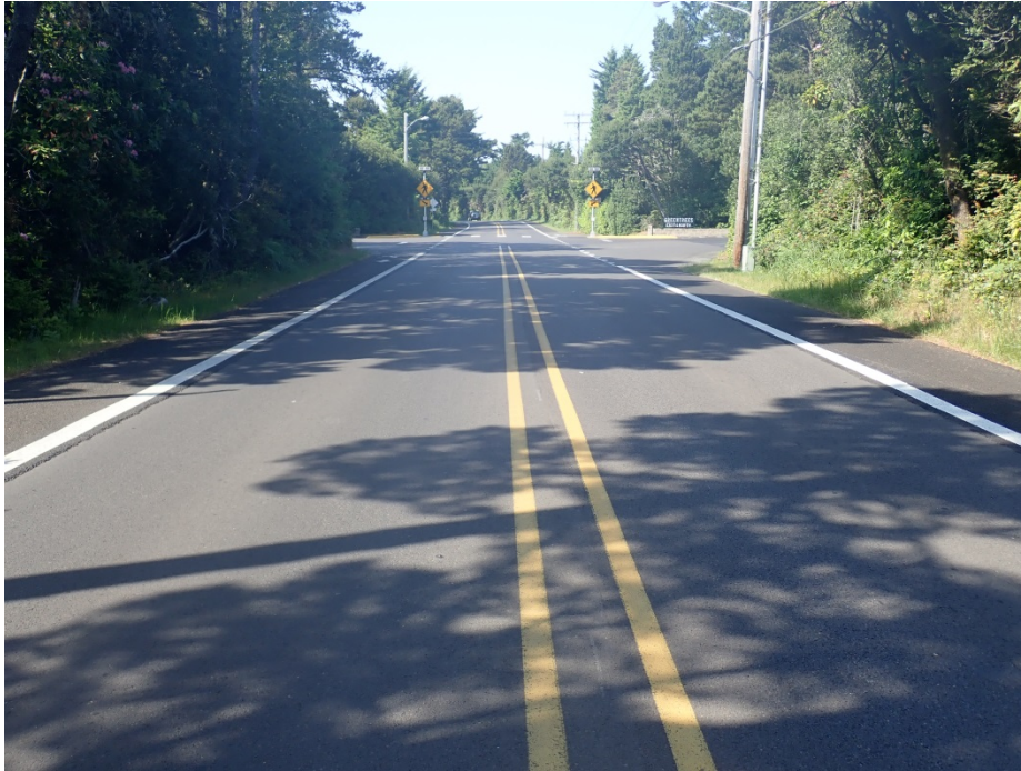
25. Looking north from 225 feet south of Green Trees / Center Road.
