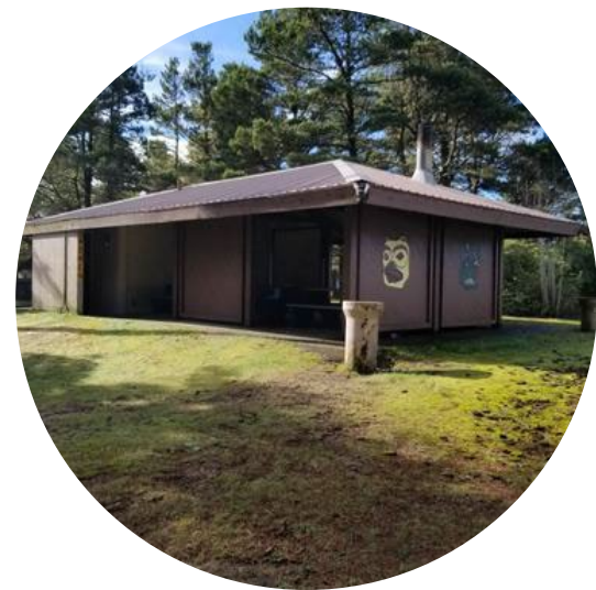
Parking lot Improvements & Picnic Shelter Construction
