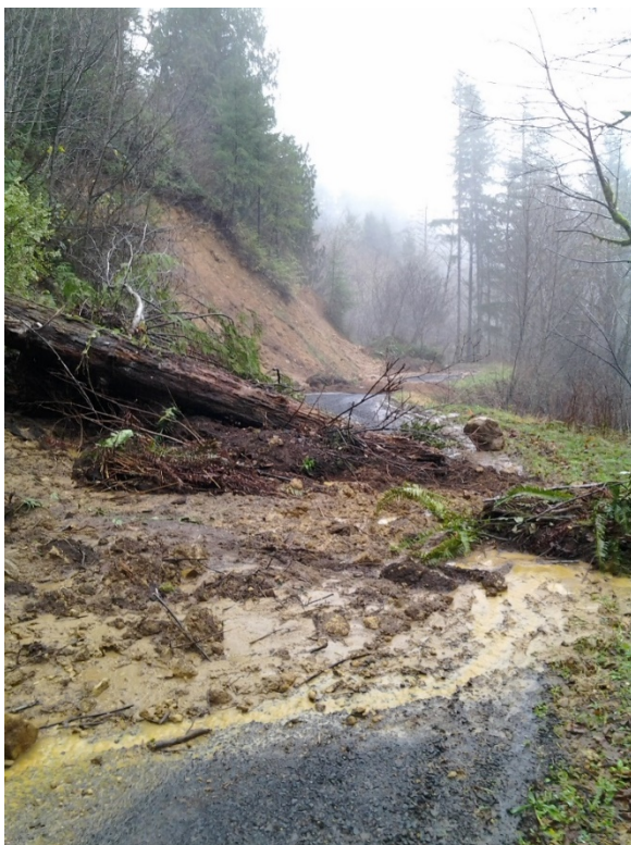
A landslide washes out a section of road near the Siuslaw River in 2014 | Photo: Lane County Public Works, Roads Division
