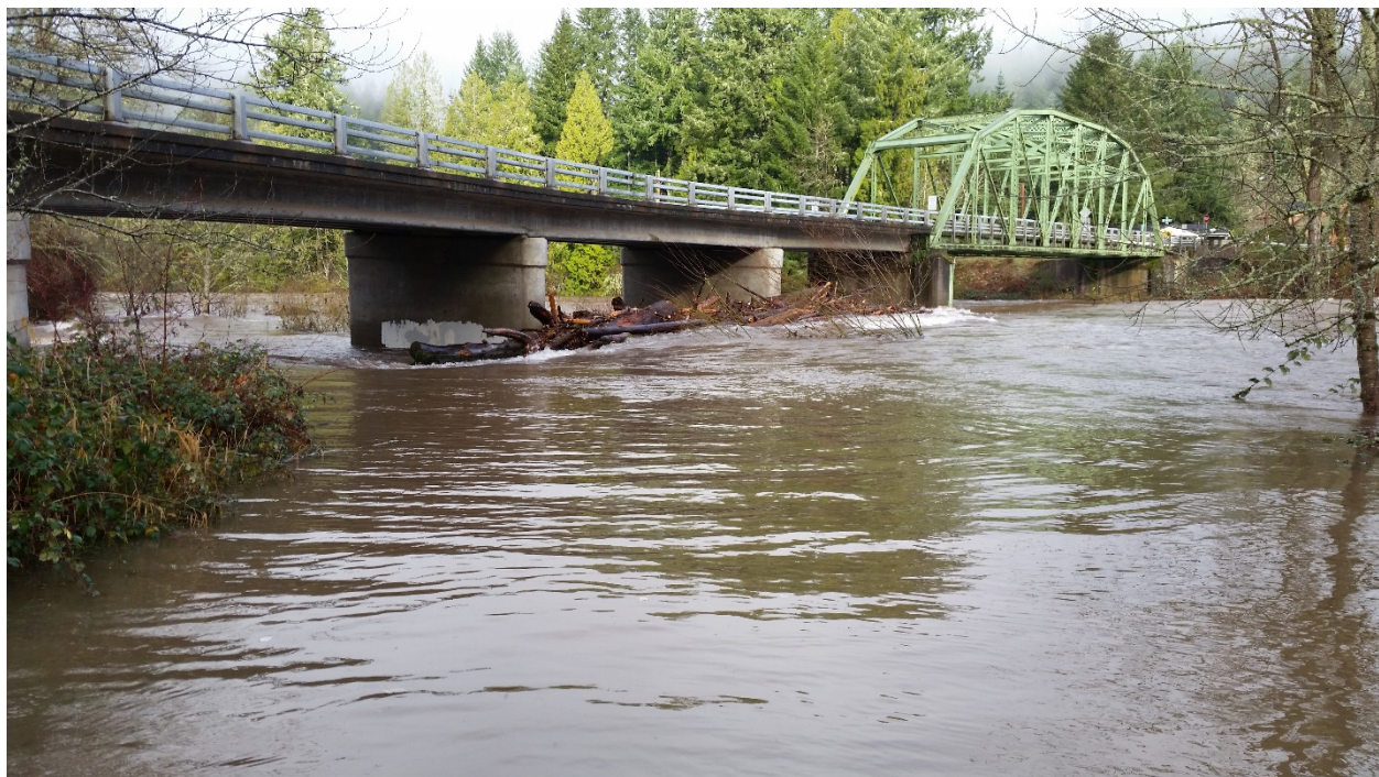
Bridge Street bridge experiencing rising waters and debris during a December 2014 event. | Photo: Lane County Public Works, Roads Division
