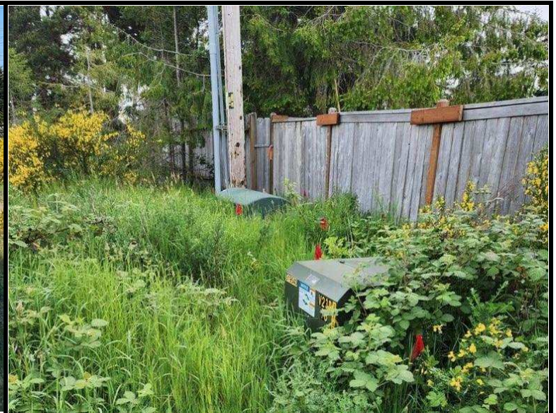
Utilities located near northeast corner
