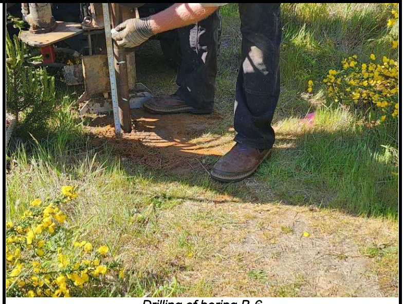
Drilling of boring B-6
