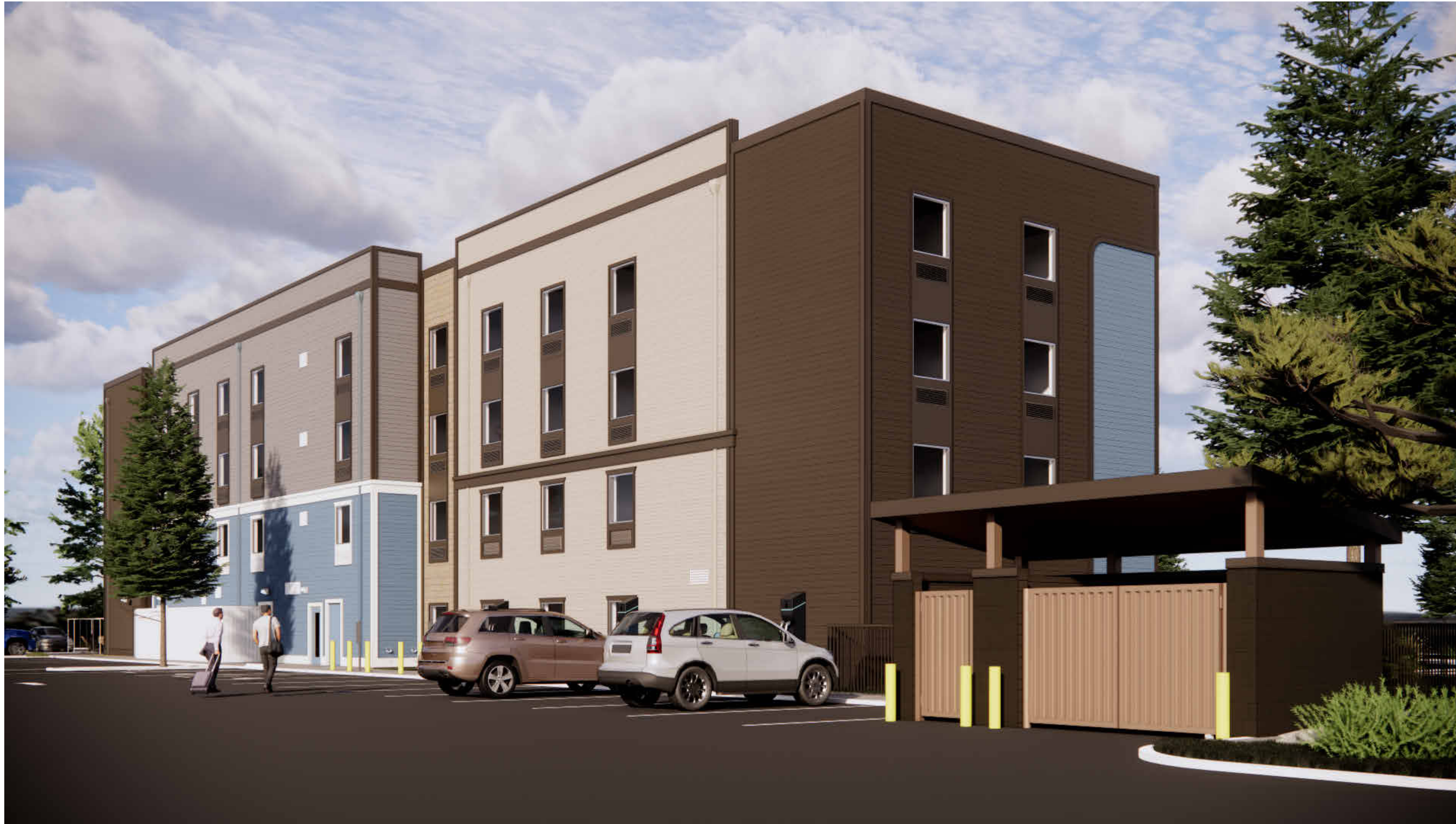
VIEW FROM NE CORNER
