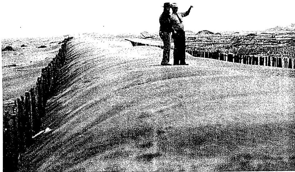
Figure 31. Warrenton Soil and Water Conservation District, Clatsop County, dune stabilization project illustrating use of sand fences to create foredune.
