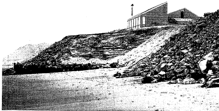
Figure 31. Homes to the south of Cape Kiwanda protected by riprap placed due to the erosion of the foredunes upon which they were being constructed (from Komar, 1978).
