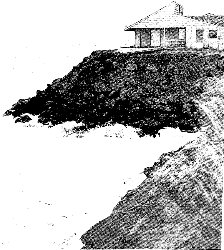
Figure 24. House left on a promontory of riprap on Siletz Spit as adjacent unprotected empty lots continued to erode (Photo by P. D. Komar, 23 January 1973).
