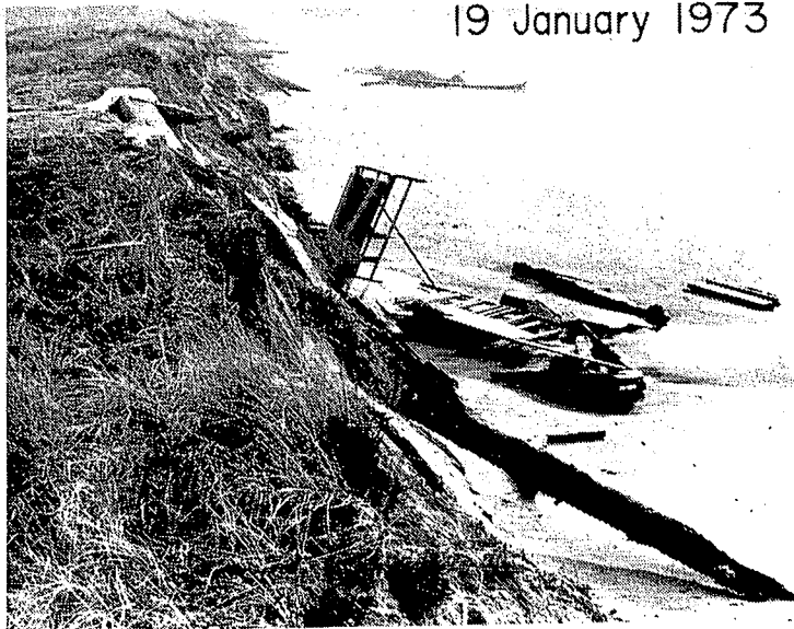
Figure 23. Destruction of house under construction on Siletz Spit due to the rapid wave erosion of the foredunes upon which the house was being built (from Komar and Rea, 1976).
