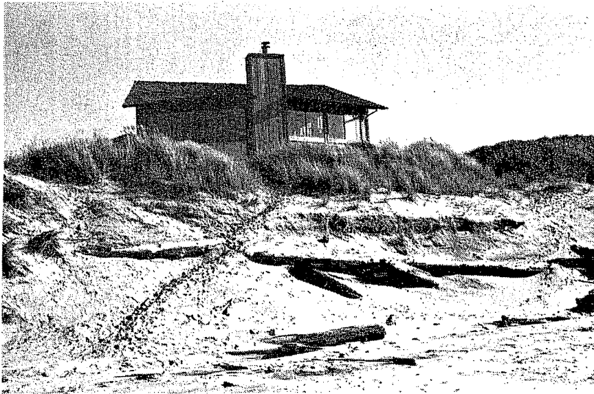
Figure 36. Homes built on Nehalem Spit in an area of active foredunes susceptible both to ocean wave attack and wind erosion.
