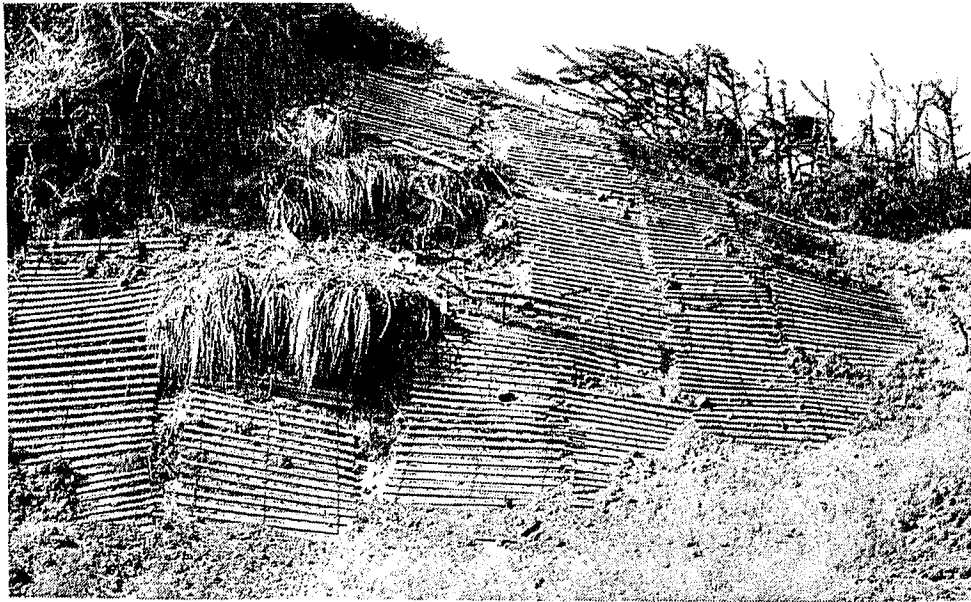
Figure 33. Snow fencing placed flat on the ground can provide temporary stabilization on cut banks, such as that performed above in Lane County, Oregon.
