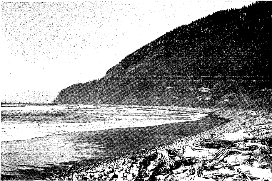
Figure 3. The beach at Neakahnie Beach with a steep cobble storm ridge of large rocks derived from the nearby basalt headland, backing an otherwise sandy beach. The cobble ridge offers protection to the coastal property.
