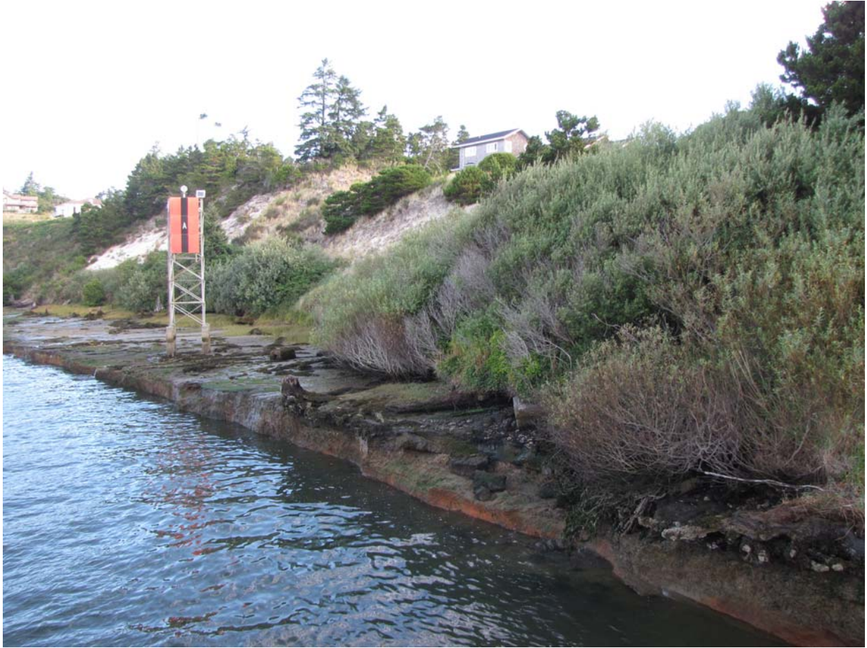
Looking downstream from walkway during low tide.
