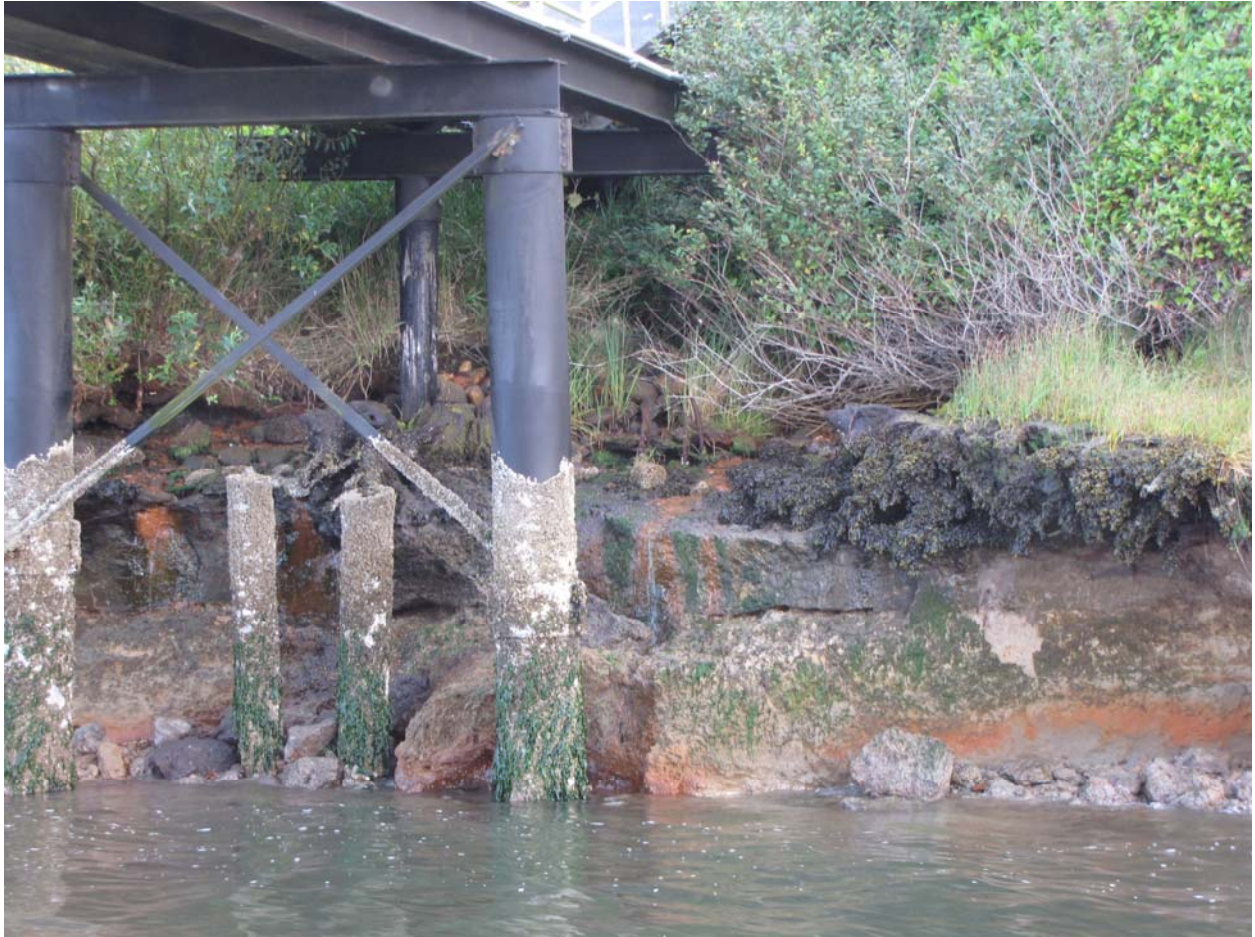
Looking east toward shoreline under base of walkway. Eroding shoreline is visible at low tide.
