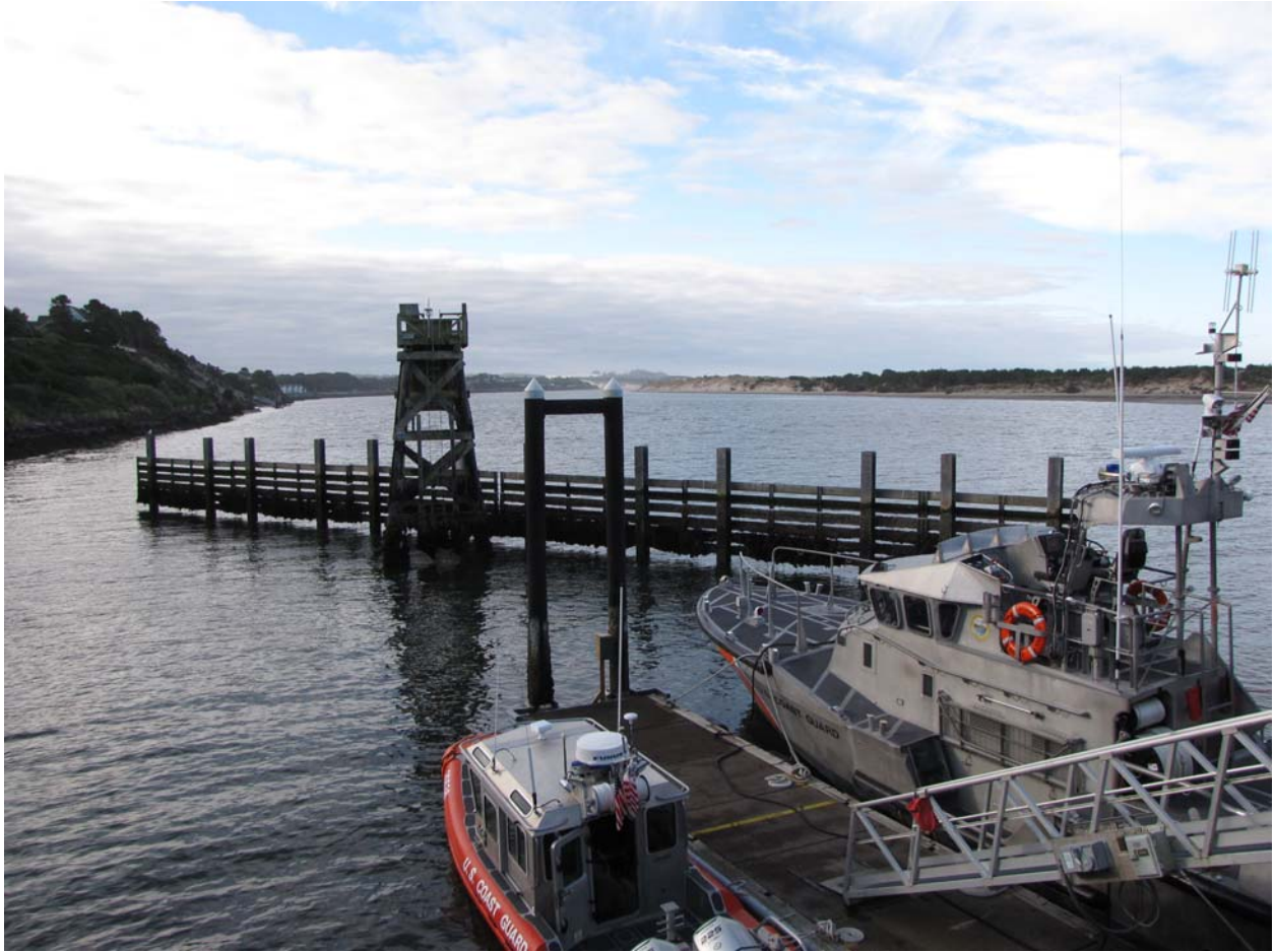
Looking south (upstream) toward debris boom.
