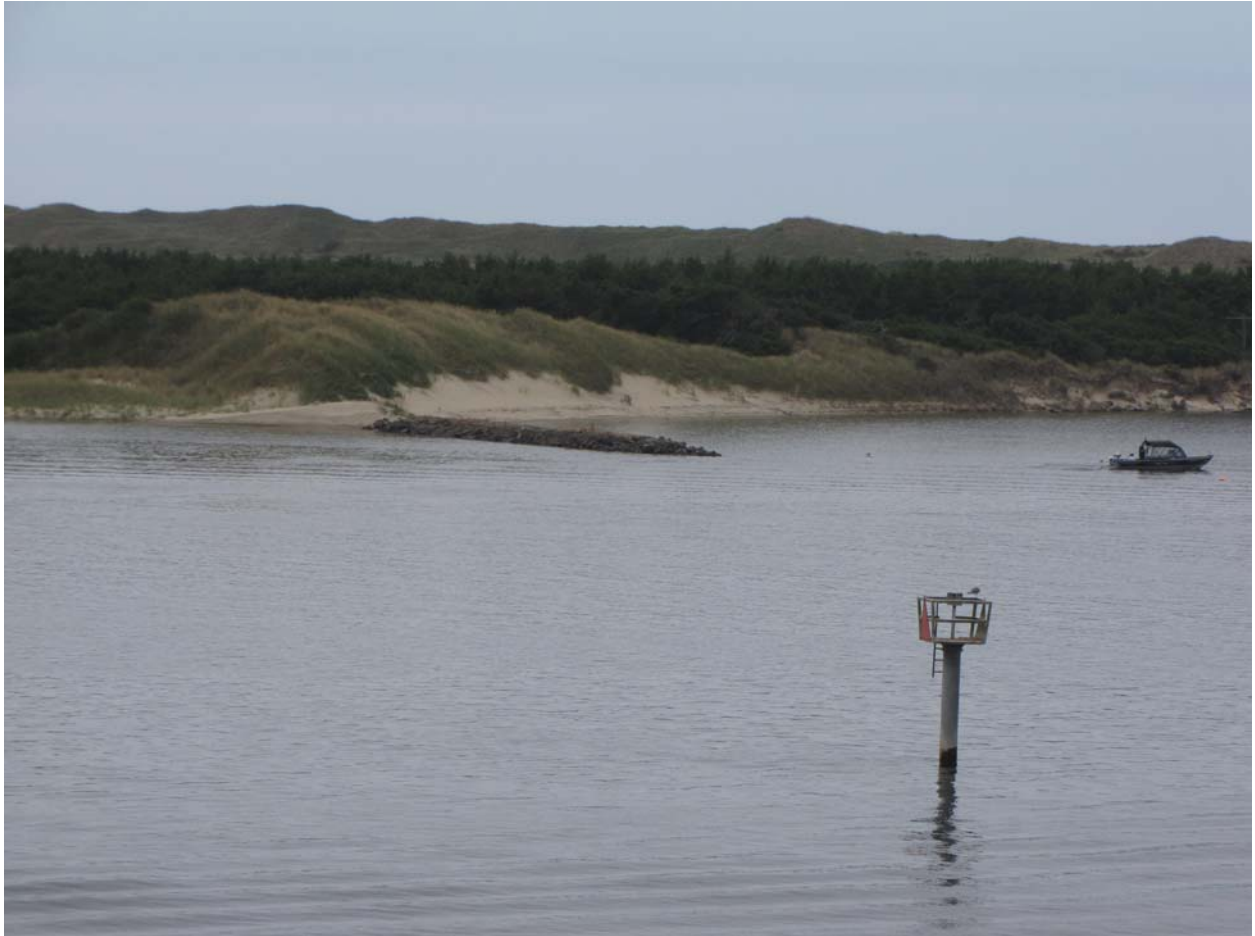
Closer view of west bank showing groins.
