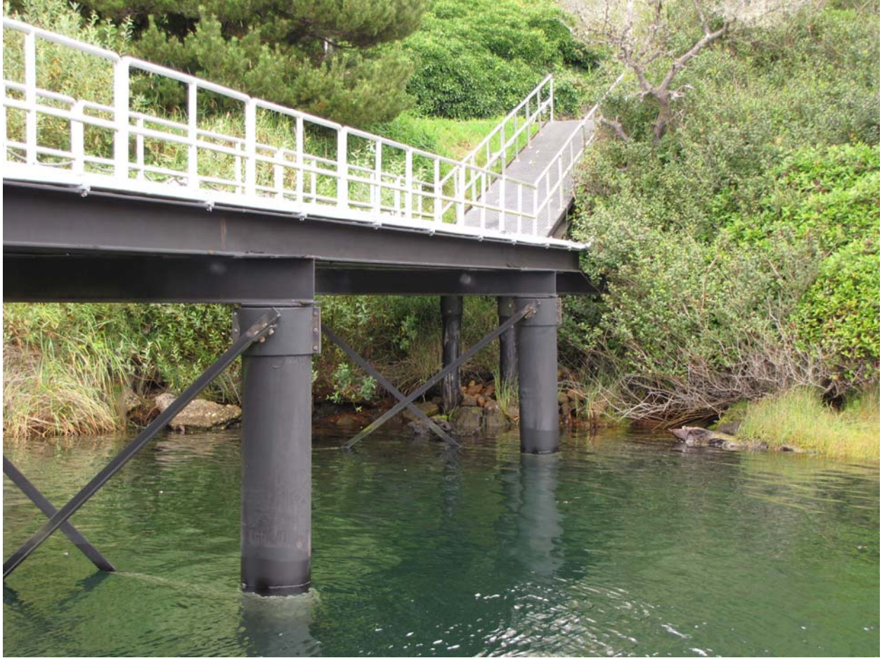
Looking east toward shoreline under base of walkway during high tide.
