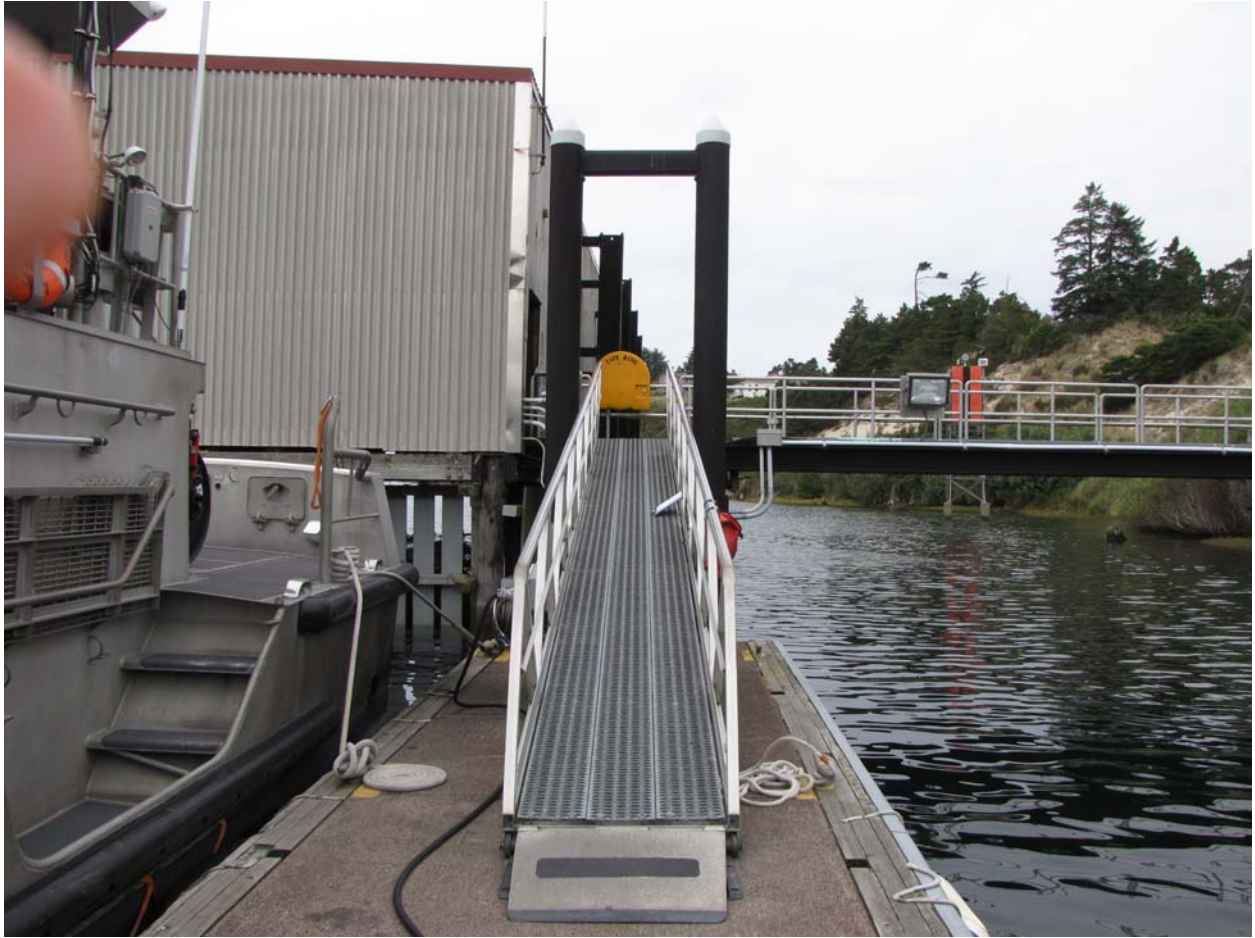
Looking north toward boathouse from dock.
