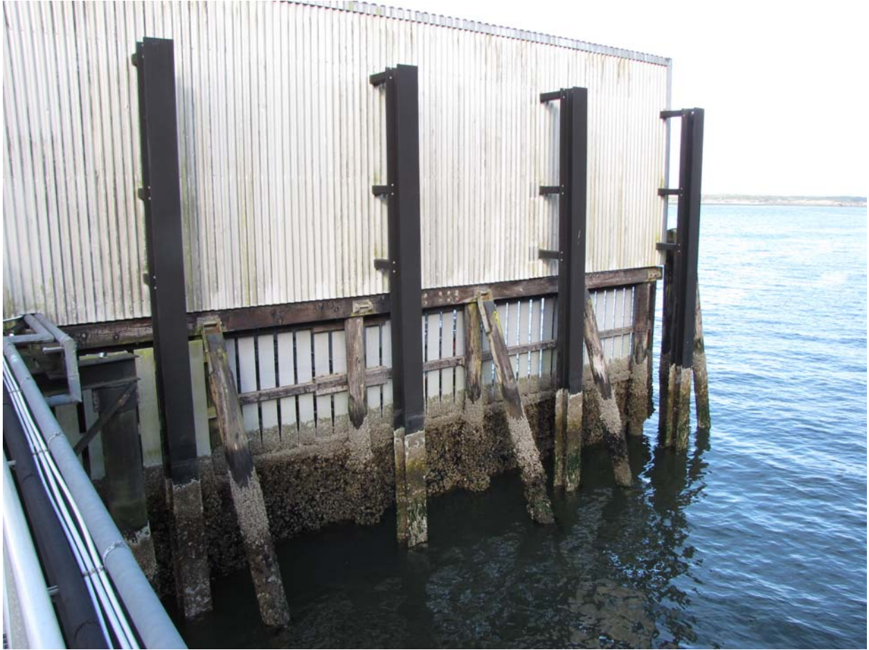
Looking west from walkway along western side of boathouse showing support beams installed in 2008.
