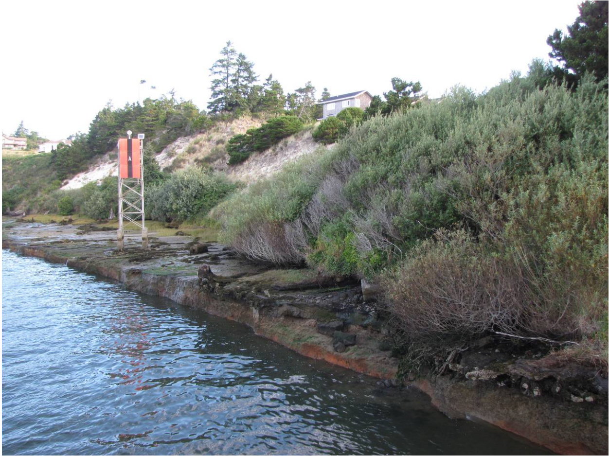
Looking downstream from walkway during low tide.
