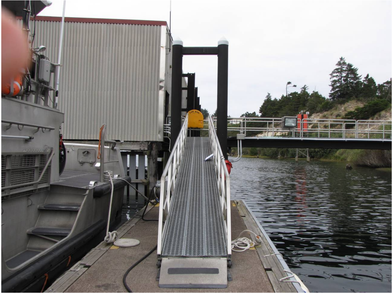
Looking north toward boathouse from dock.
