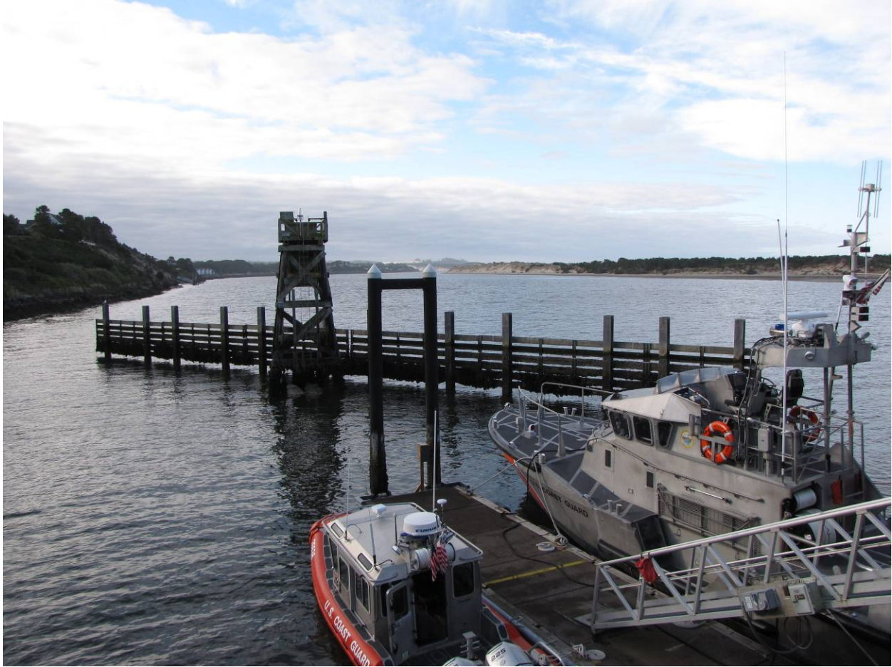
Looking south (upstream) toward debris boom.
