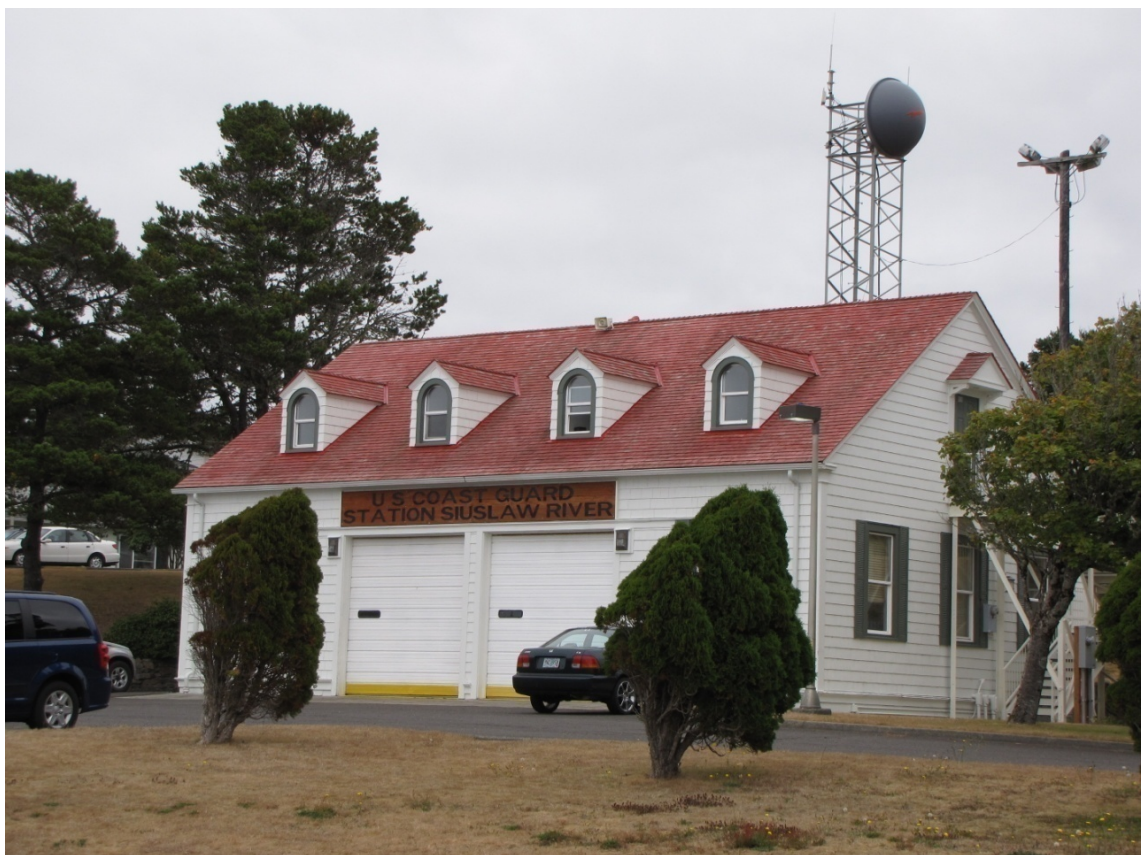
Figure 12. USCG Station Siuslaw River Equipment Building
