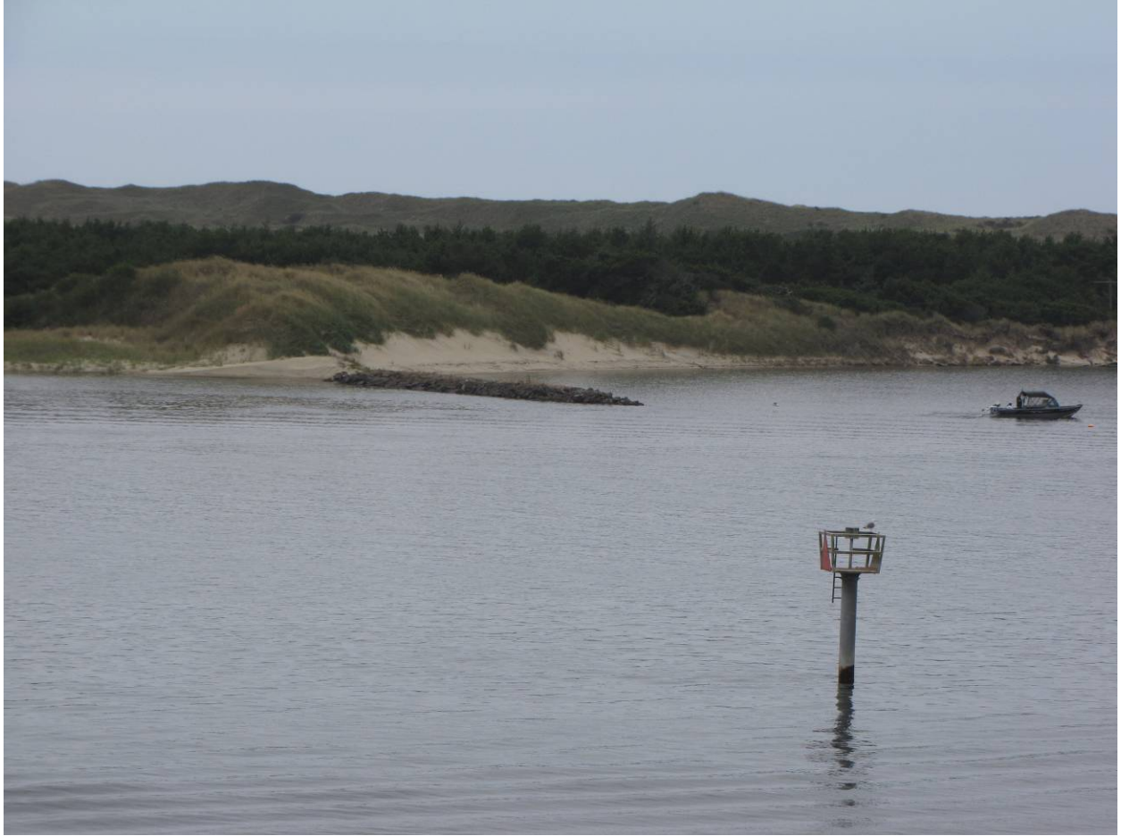
Closer view of west bank showing groins.
