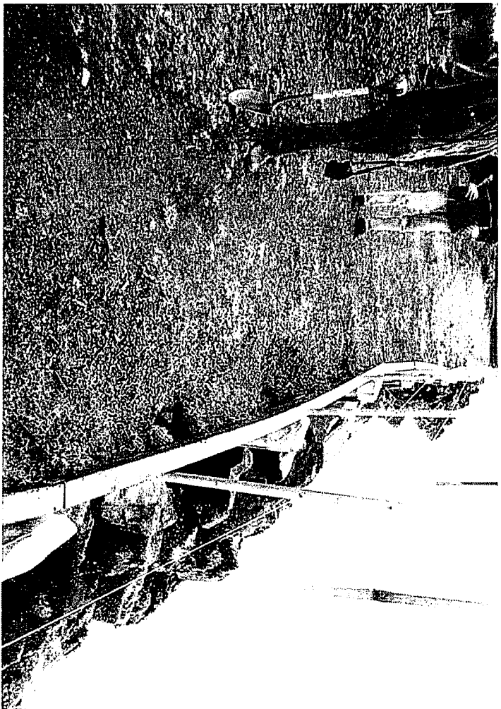
View S along seawall W of # 8/9. Note "sinkhole", bowed wall section, and leaning piles/wall.
