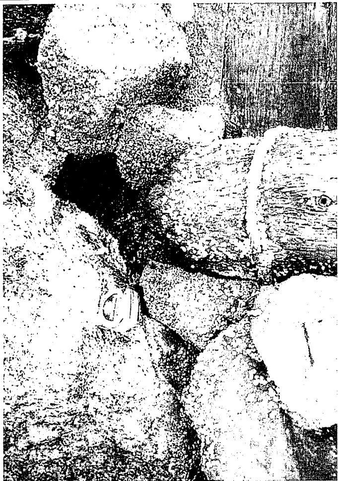
Same piling as previous photo, view E. Note lower portion completely missing. 5/30/06.
