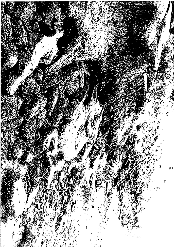
View S along bank below # 11 - 18. Note MTD exposed through older rip rap.
