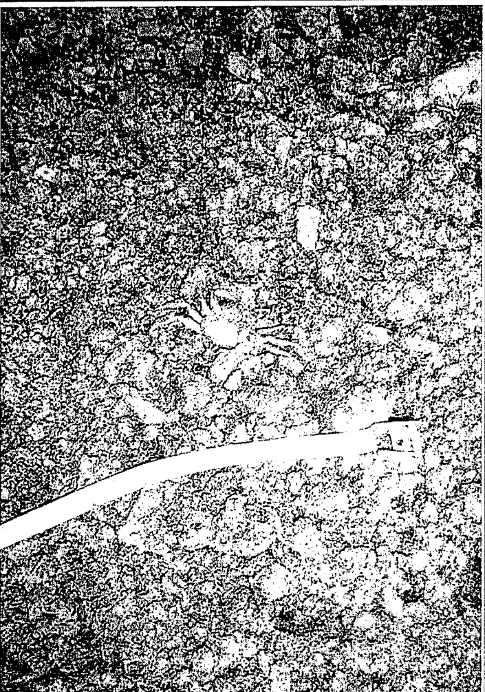
Closest view of corroded and frayed tie-back cable in previous picture. One strand may remain.
