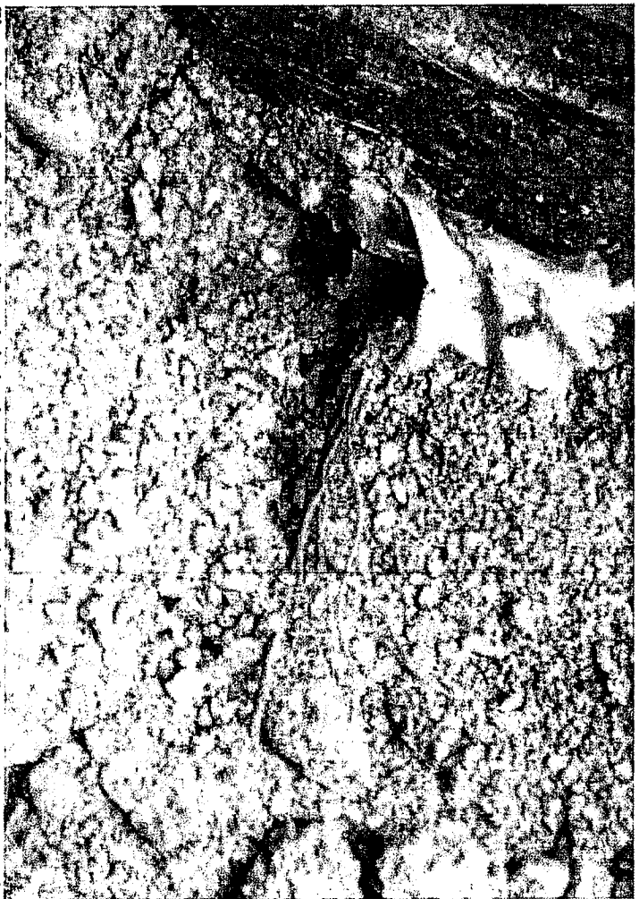
Closest view of corroded and frayed tie-back cable in previous picture. One strand may remain.
