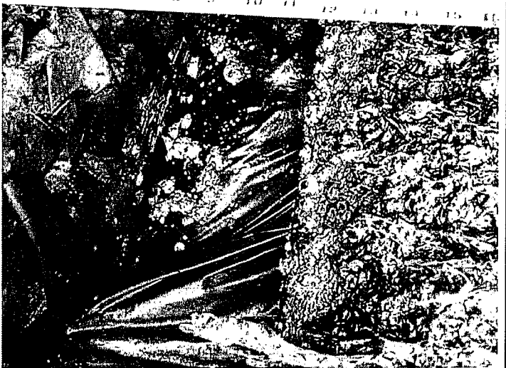
Fabric behind lagging of seawall exposed at base. 12" height to lowest lagging. View NE.
