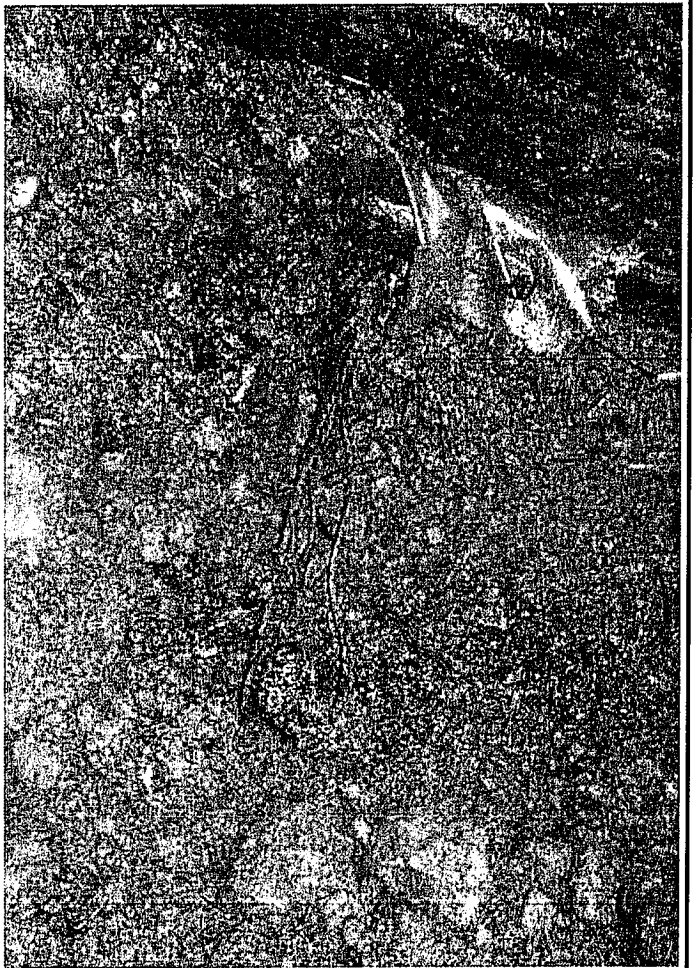
Another similar view. Cable was exposed by undermining on far side.
