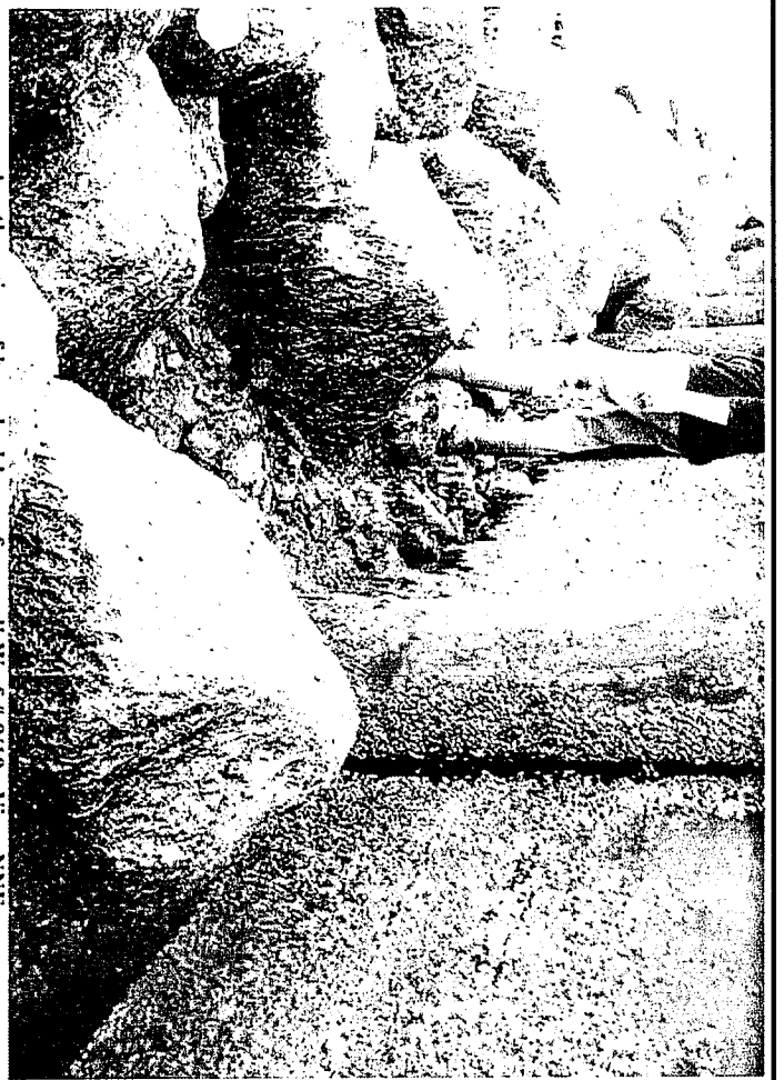
Fabric behind lagging of seawall exposed at base. 12" height to lowest lagging. View NE.
