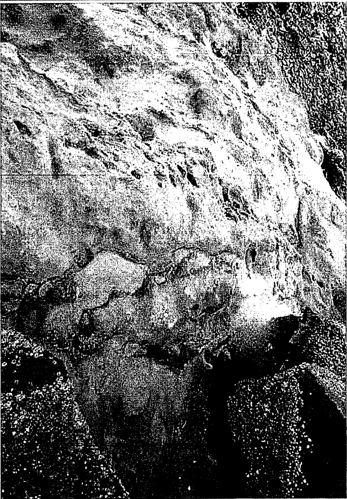
Closer view of deteriorated fabric, flowing water and sand eroded from behind fabric.
