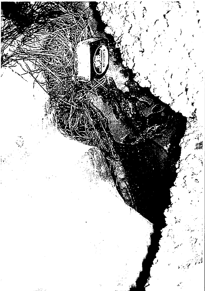
Closer view of deteriorated fabric, flowing water and sand eroded from behind fabric.
