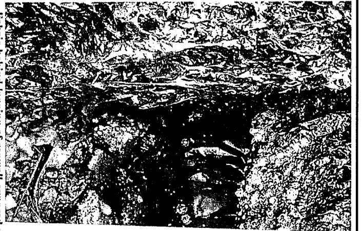
Fabric behind lagging of seawall exposed at base. 12" height to lowest lagging. View NE.
