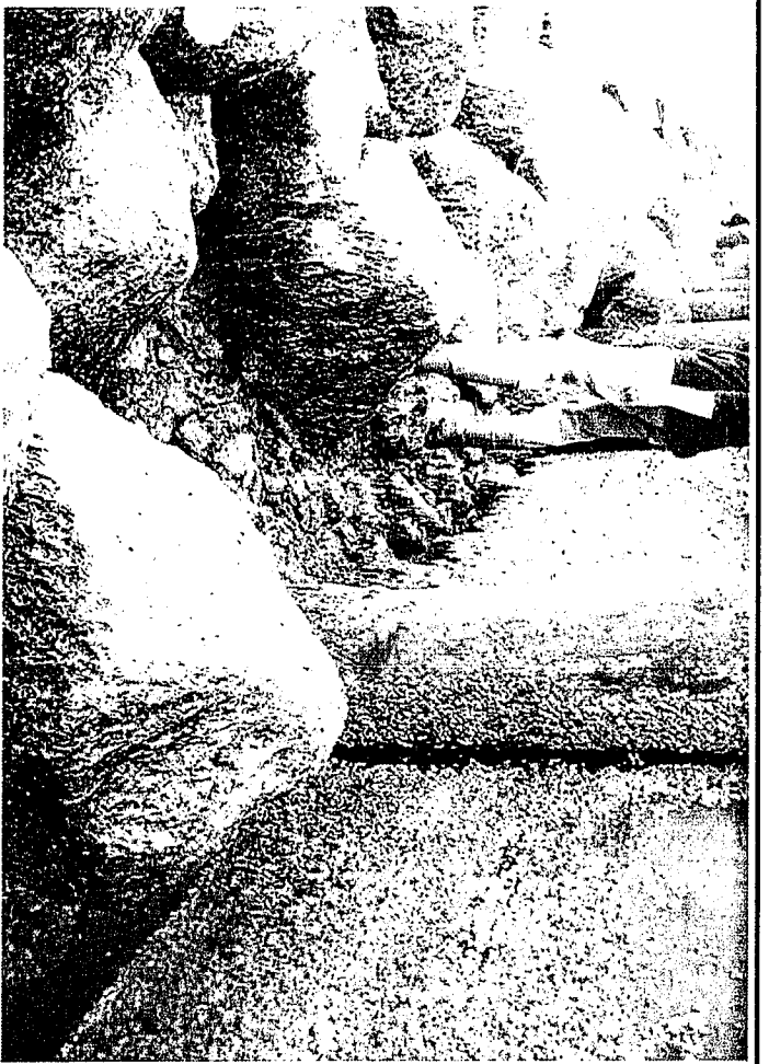
Another view of breached base of seawall W of # 9/10. View NNE.
