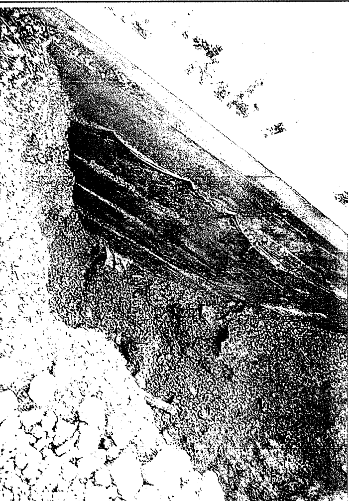
Shearing of retained soil in response to westward movement of seawall.
