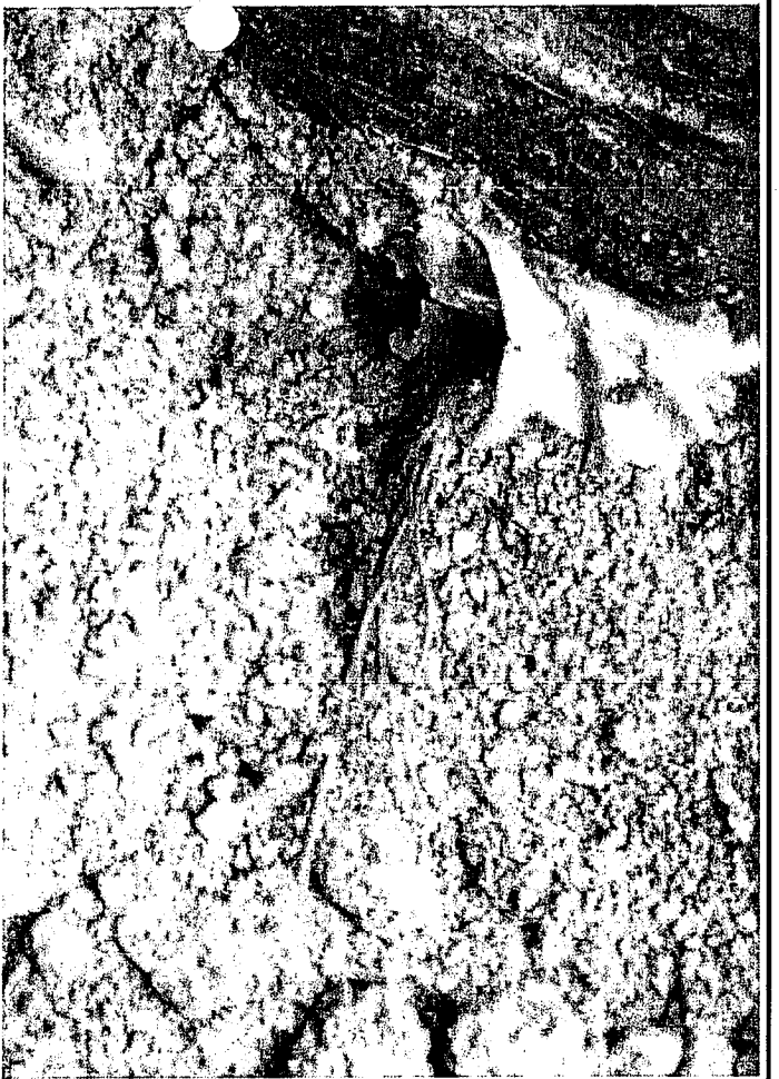
Close-up view of corroded and frayed tie-back cable in previous picture. One strand may remain.
