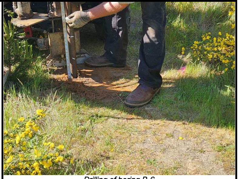
Drilling of boring B-6
