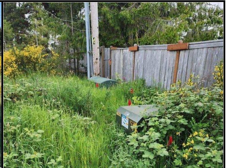
Utilities located near northeast corner
