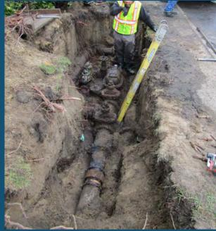
One of the early challenges was the discovery of an old metered water inter-tie connection, which required Florence Public Works crews to intervene unexpectedly. This highlighted the importance of site investigations prior to construction, as such discoveries can significantly impact project timelines and budgets. However, K&E Excavating quickly adapted to these challenges, progressing with tree trimming and utility work that laid the groundwork for further developments.
