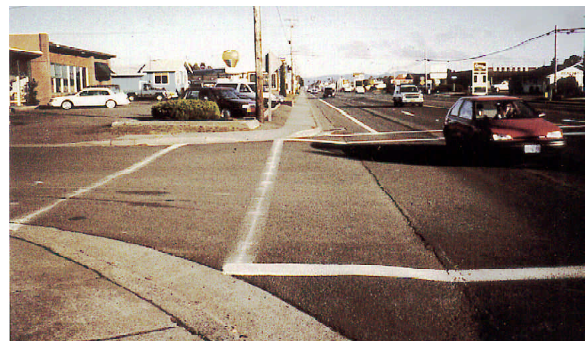
Existing Highway 101 with parking lots in front of stores
